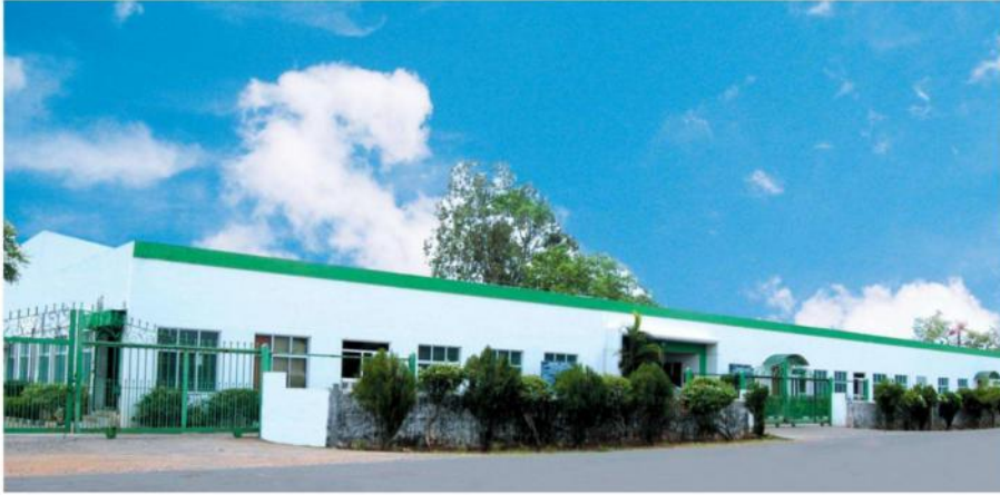
Manufacturing Plant - Chennai
